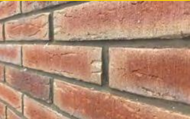
Panel bricks, splitting instead of sawing
